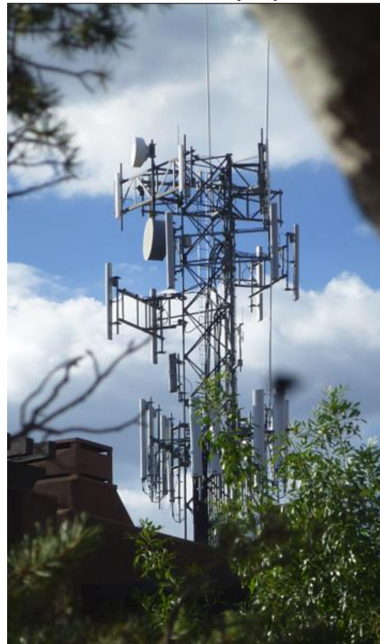
Cell tower is mostly exposed
